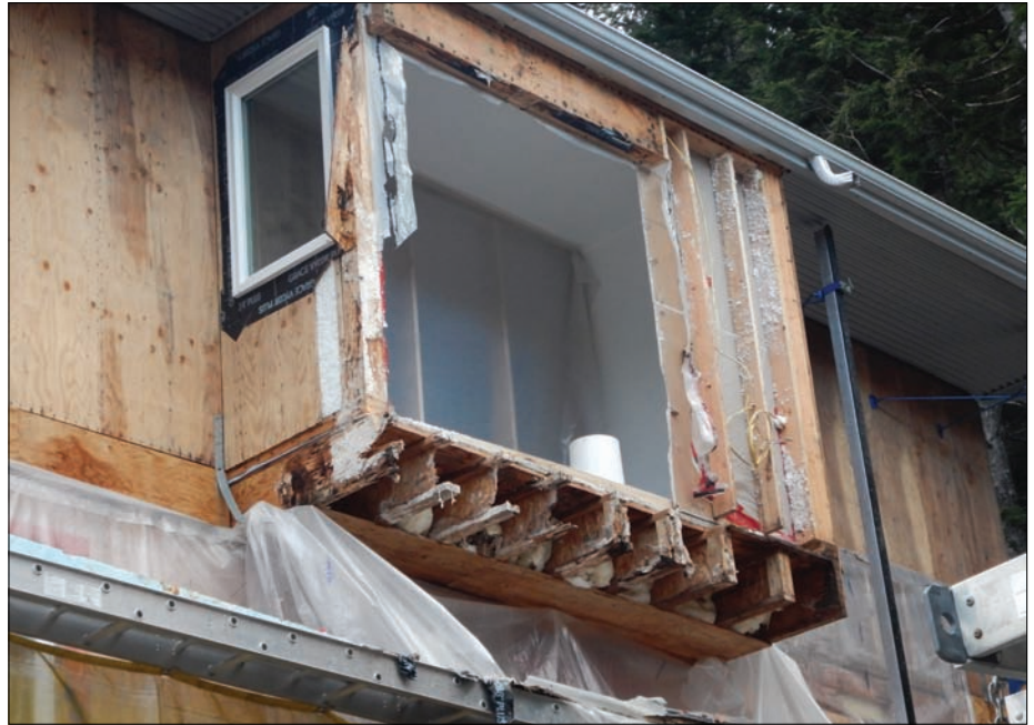
In assessing the damage to the housing units, the Coast Guard confirmed high levels of humidity, indicating a risk to human health from mold and the possibility of structural failure from rot.
